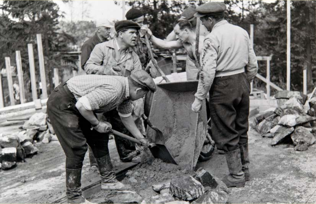
Construction work on the clubhouse of the Leppävaara workers' association, 1957. KAMU Espoo
