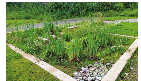
Vegetated depression designed for the detention and treatment of rainwater.
