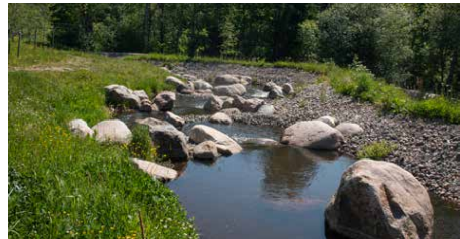
In 2020, a 190-metre-long fishway was built on the Gumbölenjoki dam, allowing migratory fish to pass the dam. Large stones have been placed in the winding channel to direct the flow of the water and create varying flow conditions. Image: Noelle Renberg
