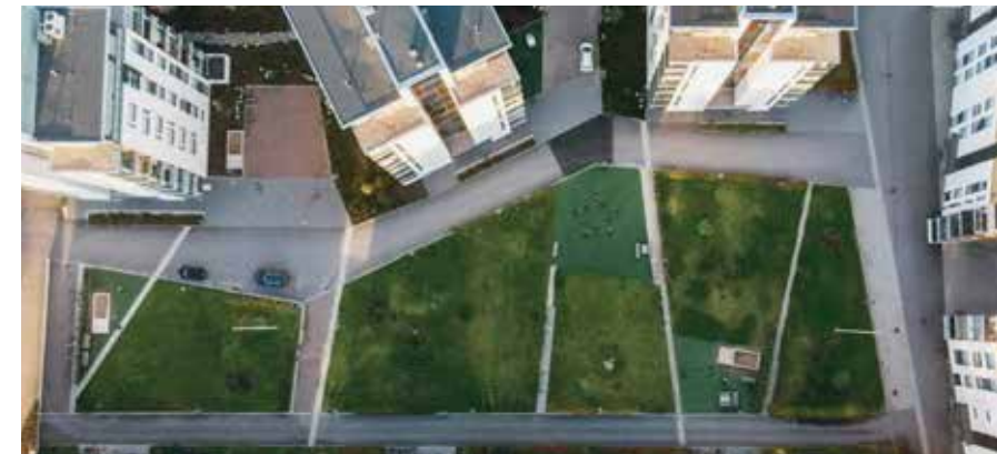
The multi-storey car parks in Revontulikortteli in Tapiola have a roof deck garden on which small trees, shrubs, dry peat and grass grow. The extensive deck garden can be seen from the surrounding buildings and provides a place for activities such as playing ball in an area of open grass. Image: Pyry Kantonen
